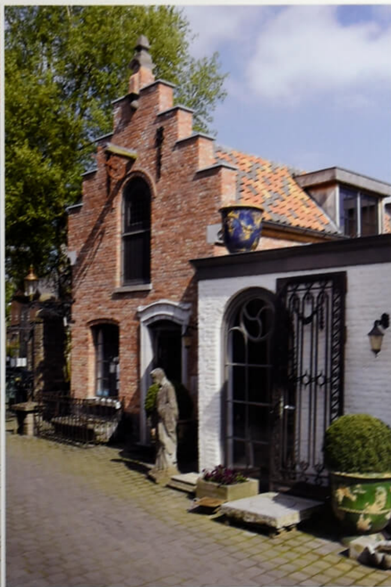
A newly built old-style exterior wall with old bricks, wall clamps and other details. A bluestone door surround and old-fashioned street lighting.
